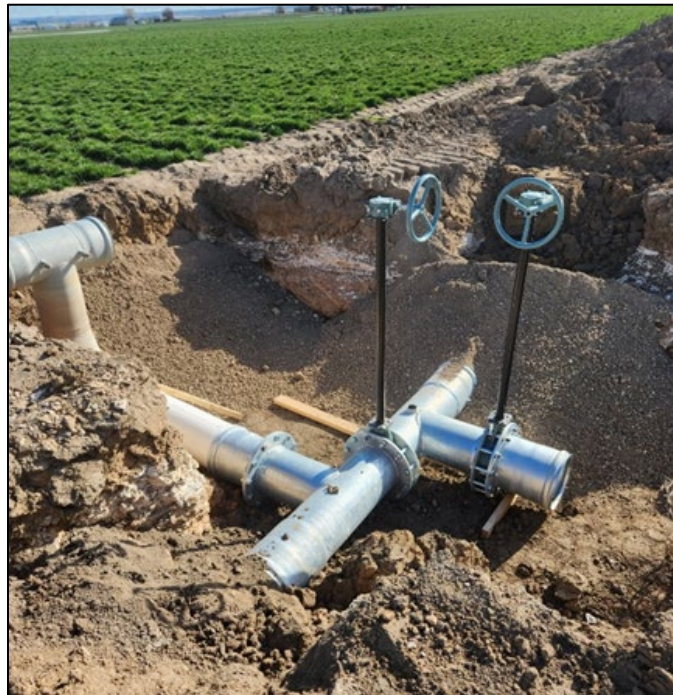
Connecting new pivot to buried mainline
