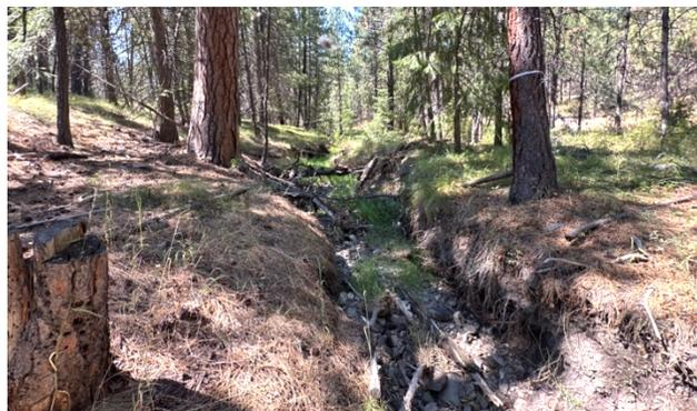
Incised section of Dick Creek currently undergoing channel fill and large wood placement, as part of Upper Trout Creek Tributary Rehab project with FS partners. Incised channel is being filled with natural materials borrowed from adjacent decommissioned road.
